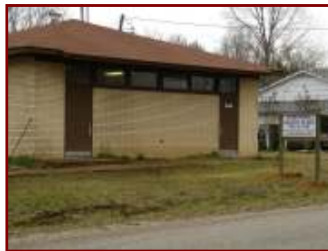
CCMC Rural Health Clinic in Weir
